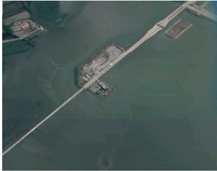
Figure 2. The Sightings of the Case Study Port Terminal
