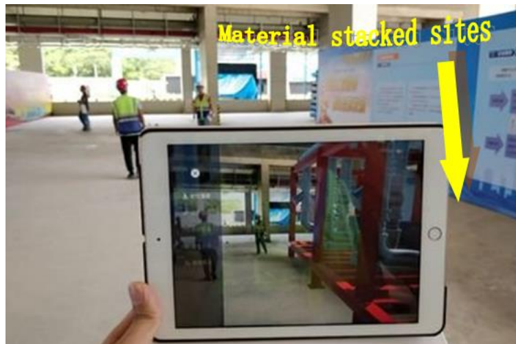
Fig.2. Material stacking operation diagram based on AR technology
