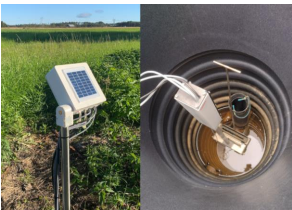
Fig 2. Prototype of controlled well installed to test area.
