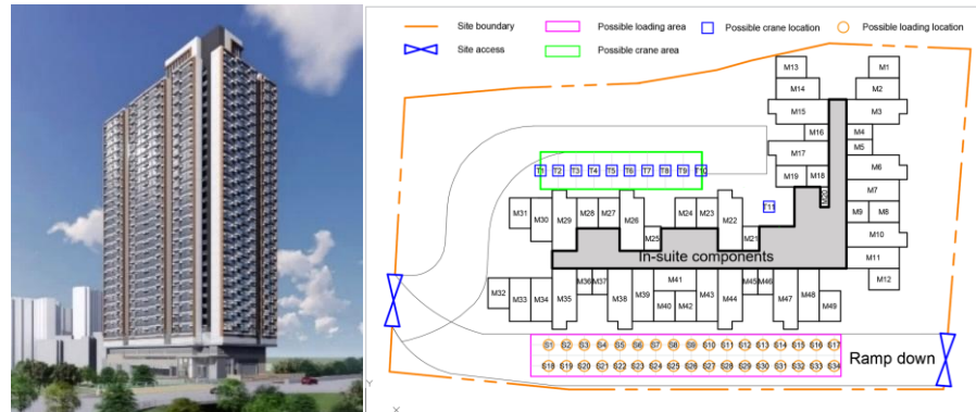
Figure 3: The exterior view of the construction site and site layout scheme
